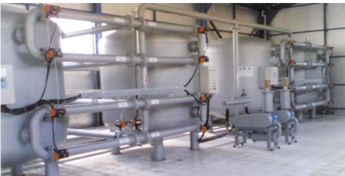
19. Sand Filter and Activated Carbon Filter / Kum Filtresi ve Aktif Karbon Filtresi
