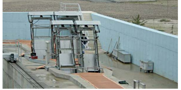
2. Manual and Mechanical Screens / Manuel ve Mekanik Izgaralar
