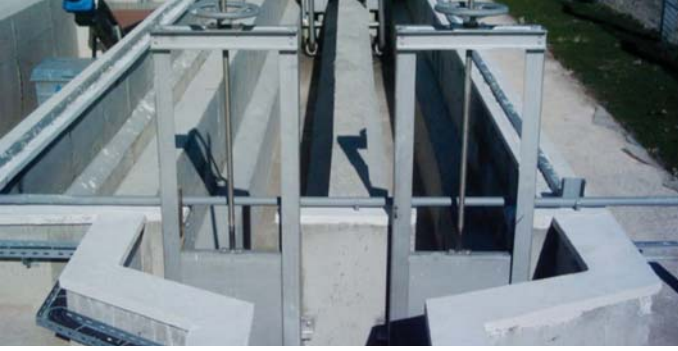
1. Penstock/ Sluice Gate / Stop Log / Kapak
