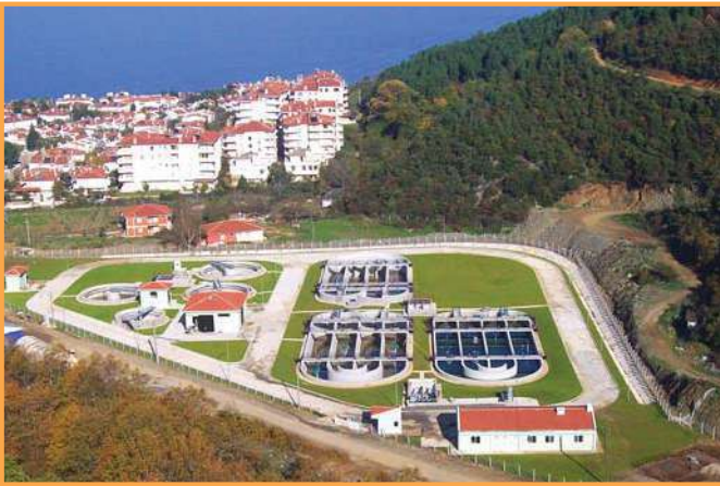
Esenköy Atıksu Arıtma Tesisi / YALOVA Esenköy Waste Water Treatment Plant / YALOVA
