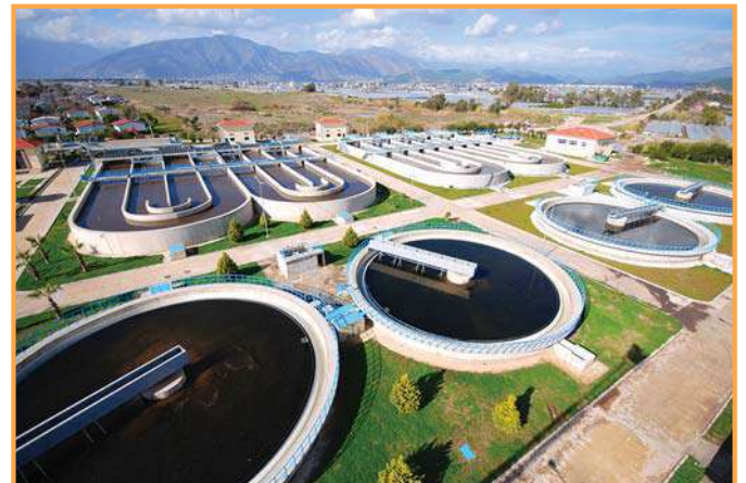
Kumluca Atıksu Arıtma Tesisi / ANTALYA Kumluca Waste Water Treatment Plant / ANTALYA
