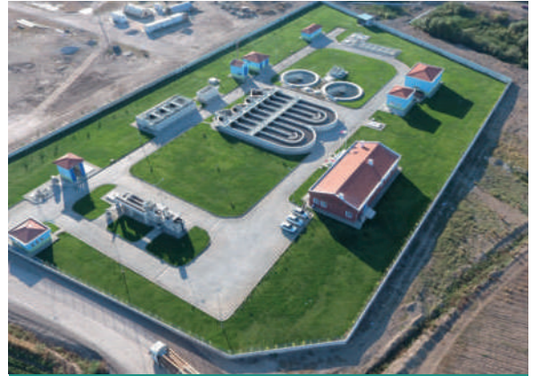
BİĞADİÇ (BALIKESİR) ATIKSU ARITMA TESİSİ BIGADIC (BALIKESİR) WASTEWATER TREATMENT PLANT
