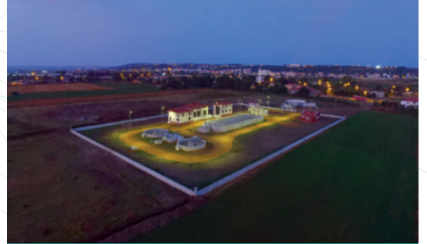
İPSALA (EDİRNE) ATIKSU ARITMA TESİSİ İPSALA (EDİRNE) WASTEWATER TREATMENT PLANT
