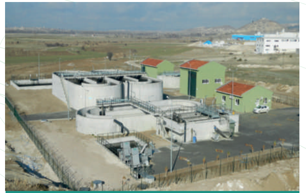
KÜTAHYA OSB ENDÜSTRİYEL ATIKSU ARITMA TESİSİ KÜTAHYA ORGANIZED INDUSTRIAL ZONE INDUSTRIAL WASTEWATER TREATMENT PLANT
