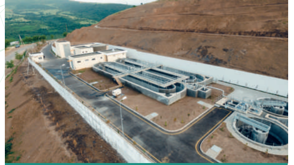
LERİK (AZERBAIJAN) ATIKSU ARITMA TESİSİ LERİK (AZERBAIJAN) WASTEWATER TREATMENT PLANT
