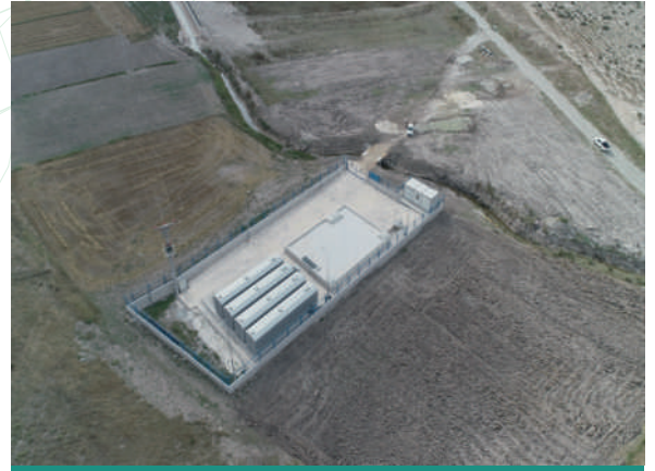
KIRKA (ESKİŞEHİR) PAKET ARITMA TESİSİ KIRKA (ESKİŞEHİR) PACKAGE TREATMENT PLANT
