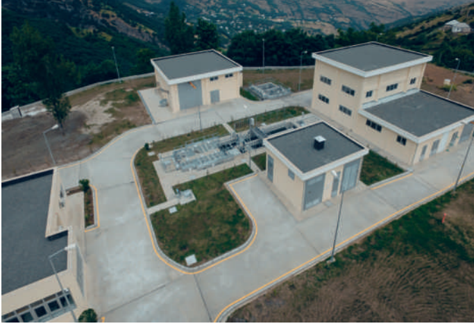
İÇME SUYU ARITMA TESİSLERİ Potable Water Treatment Plants
