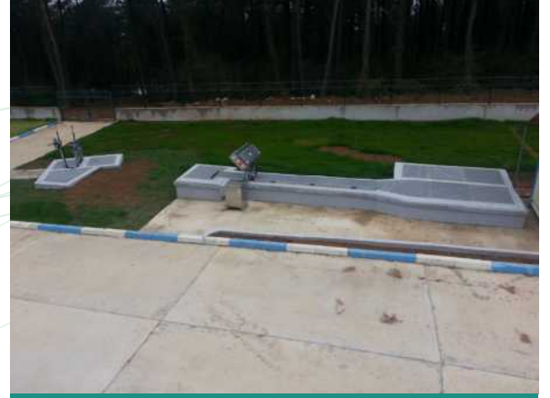
KOCAELİ (CEBECİ) ATIKSU ARITMA TESİSİ KOCAELİ (CEBECİ) WASTEWATER TREATMENT PLANT
