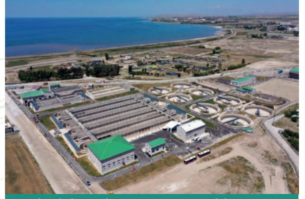
VAN İLERİ BİYOLOJİK ATIKSU ARITMA TESİSİ VAN CENTRAL ADVANCED BIOLOGICAL WASTEWATER TREATMENT PLANT
