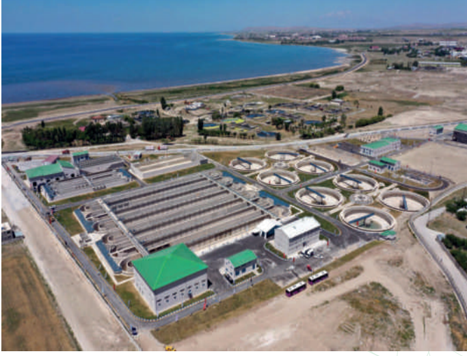
ATIKSU ARITMA TESİSLERİ Wastewater Treatment Plants
