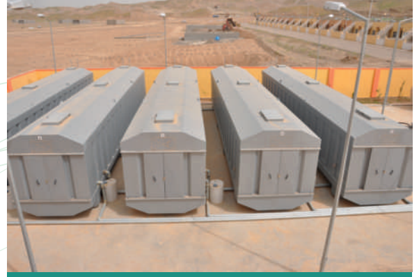
KERKÜK (İRAK) PAKET ARITMA TESİSİ KIRKUK (IRAQ) PACKAGE TREATMENT PLANT
