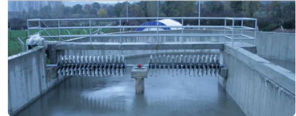
Yatay Milli Aerator | Horizontal Shaft Aerator
